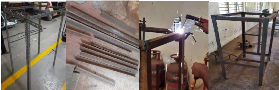
Fig 4 (a)Dummy Frame ,(b)L-Channel for Main Frame, (c) Arc Welding,(d)Main Frame
